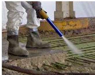
Concrete Repair & Restoration
