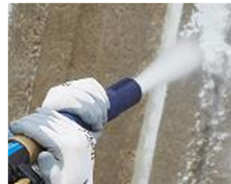
Concrete Surface Prep
