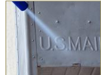
Steel Surface Prep
