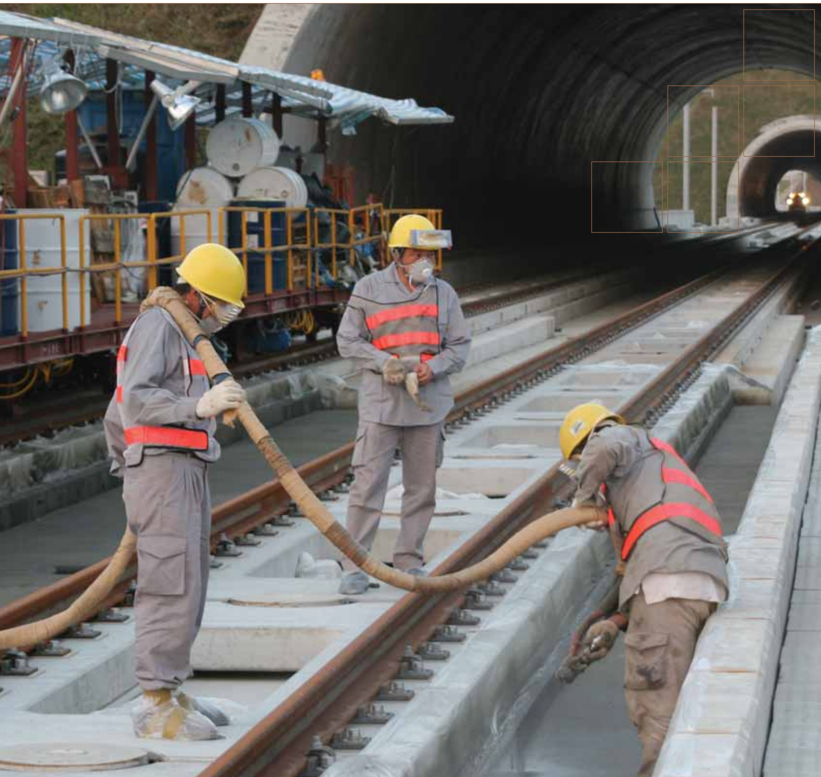
Graco's Reactor™ plural component proportioner is used to spray polyurea sealant to high-speed rail system in Taiwan
