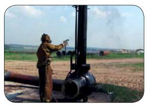
Spraying protective coatings on oil pipelines both above and below ground in Russia
