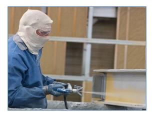
Graco XM PFP Plural-Component Sprayer
